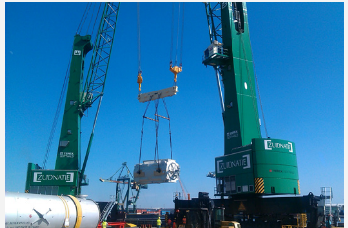
Tandem crane operation
