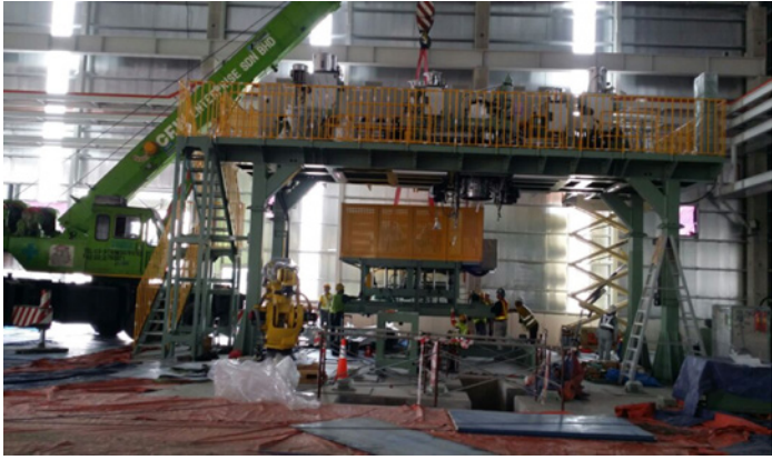
Molding Machine Installation job
