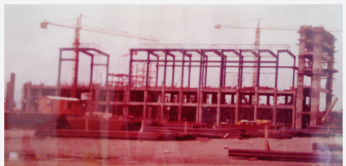
Paper machine building being erected in Puerto Dejada Colombia 1983
