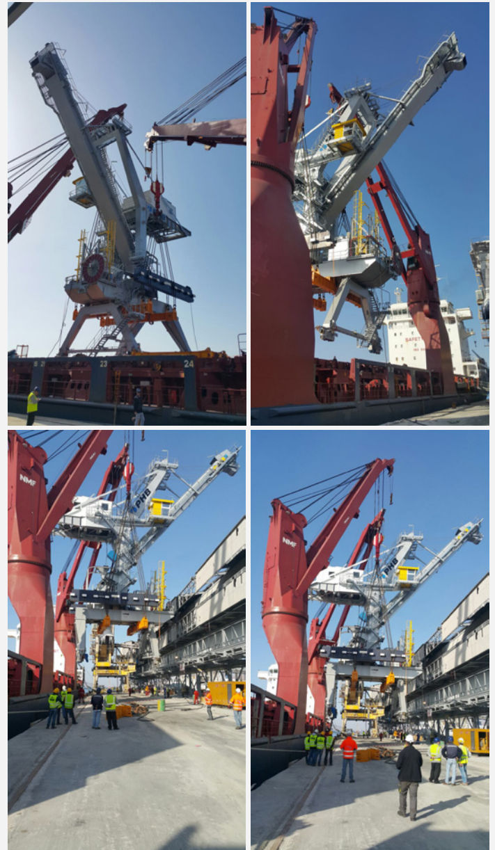
Discharging from Atlantic Winter – Aqaba, Jordan
