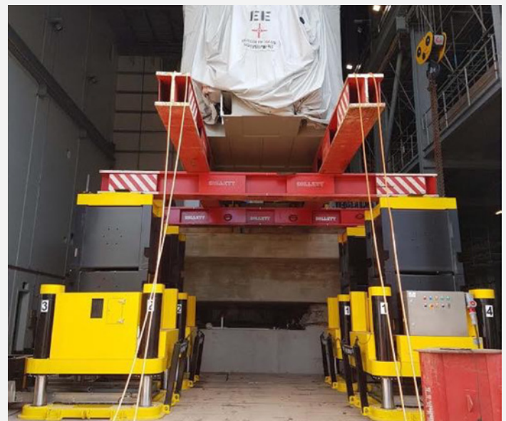
The Jack-Up system lifted the plant equipment to a height of 4.5m
