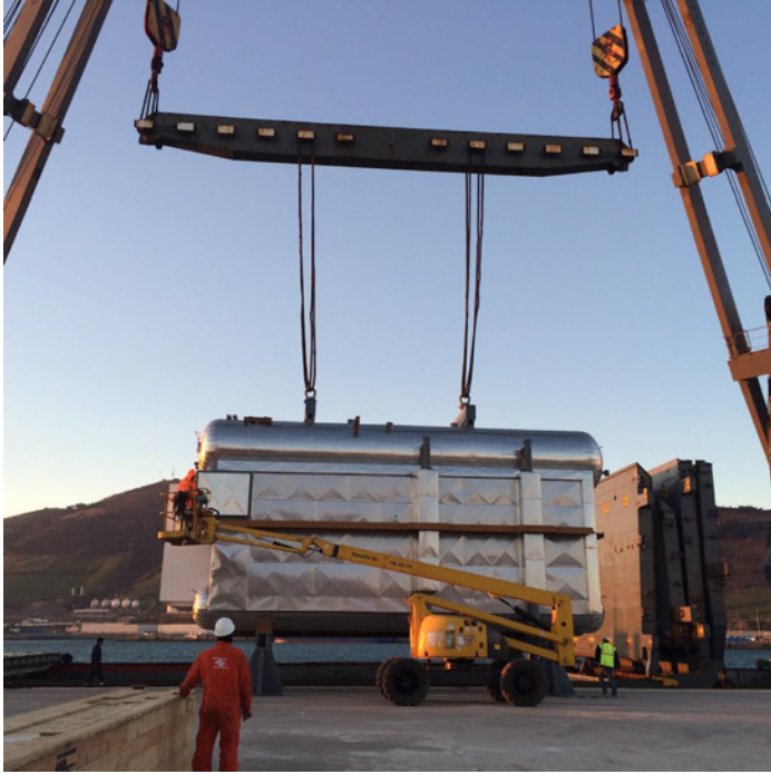
Ethilen-Boiler shipment (237mt)
