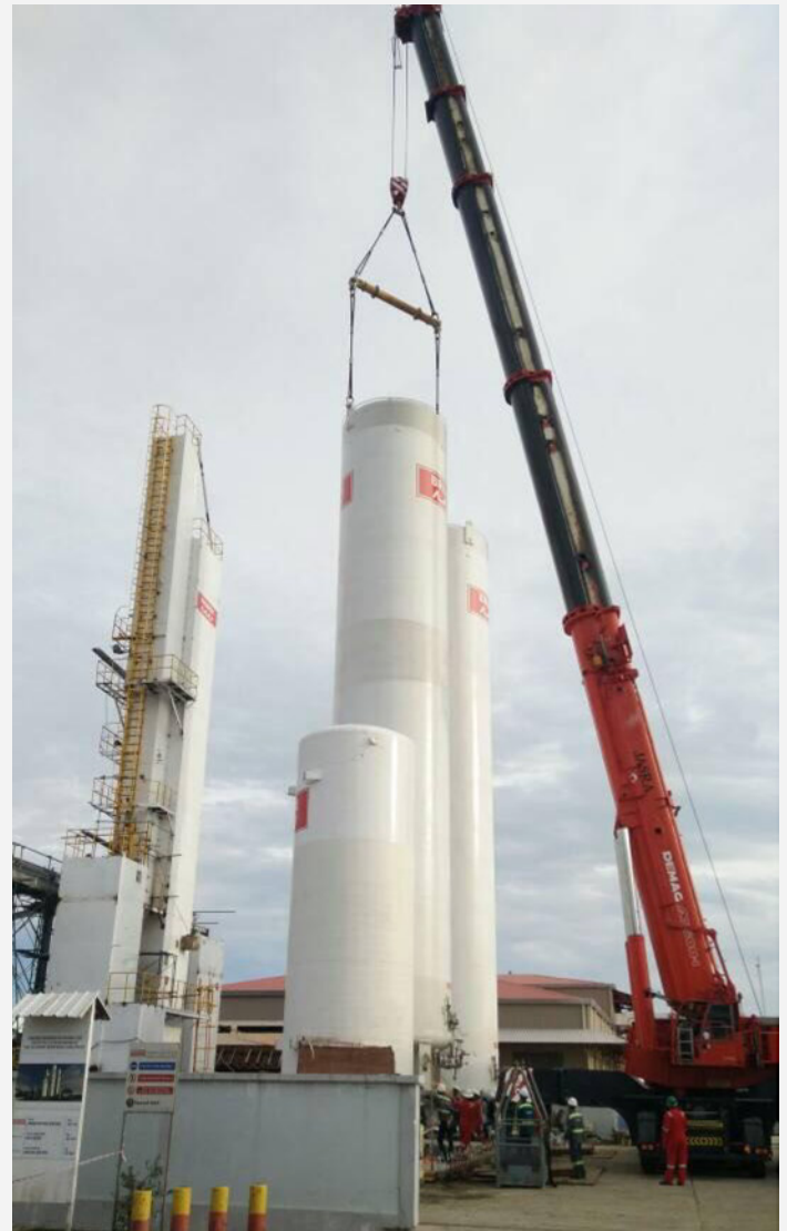
Lifitng & transpotation of LIN Tanks
