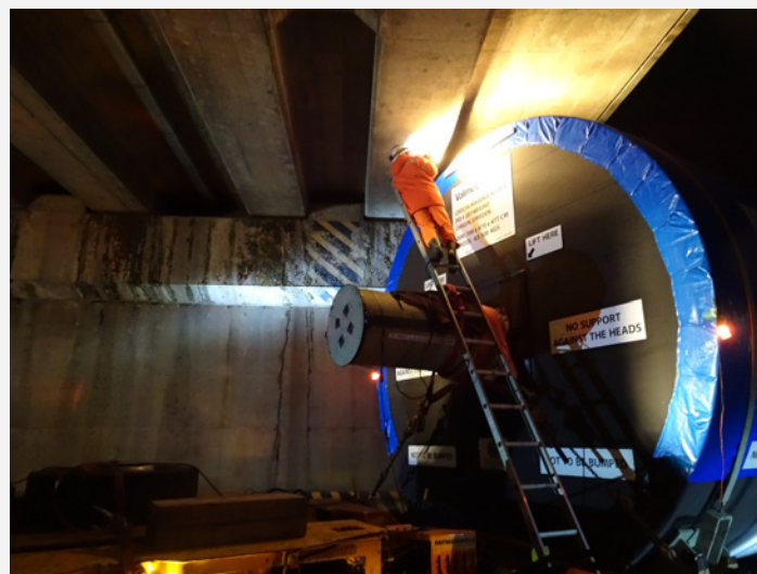
83.1 m/477 cm high Yankee passing under an 486 cm high Shinkansen (Bullet Train) elevated railway in the middle of the night on 18/Jan, 2018
